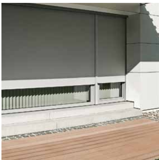
Combination of exterior heat protection and interior glare protection.
